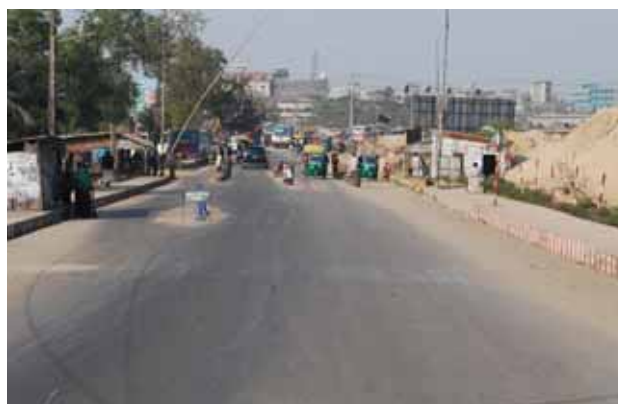
Pic. 4-29 Karnaphuli Bridge Approach Road.
